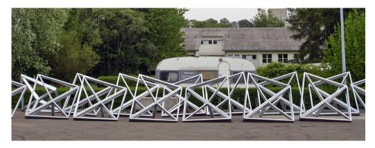
Figure 9 Fifteen galvanized roof frames waiting on the ETH campus for assembly
